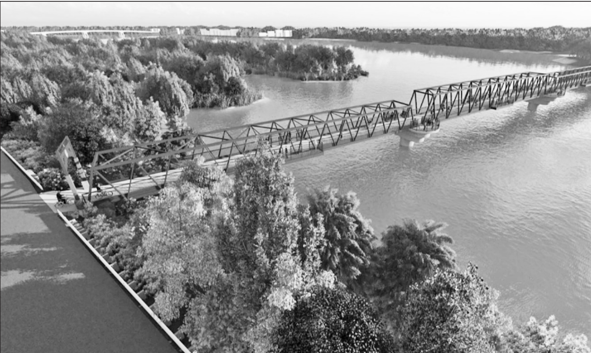
The future Wisconsin River recreation bridge, a three-span concrete and steel structure, wil feature viewing platforms and fishing spots, providing scenic views for trail users.
