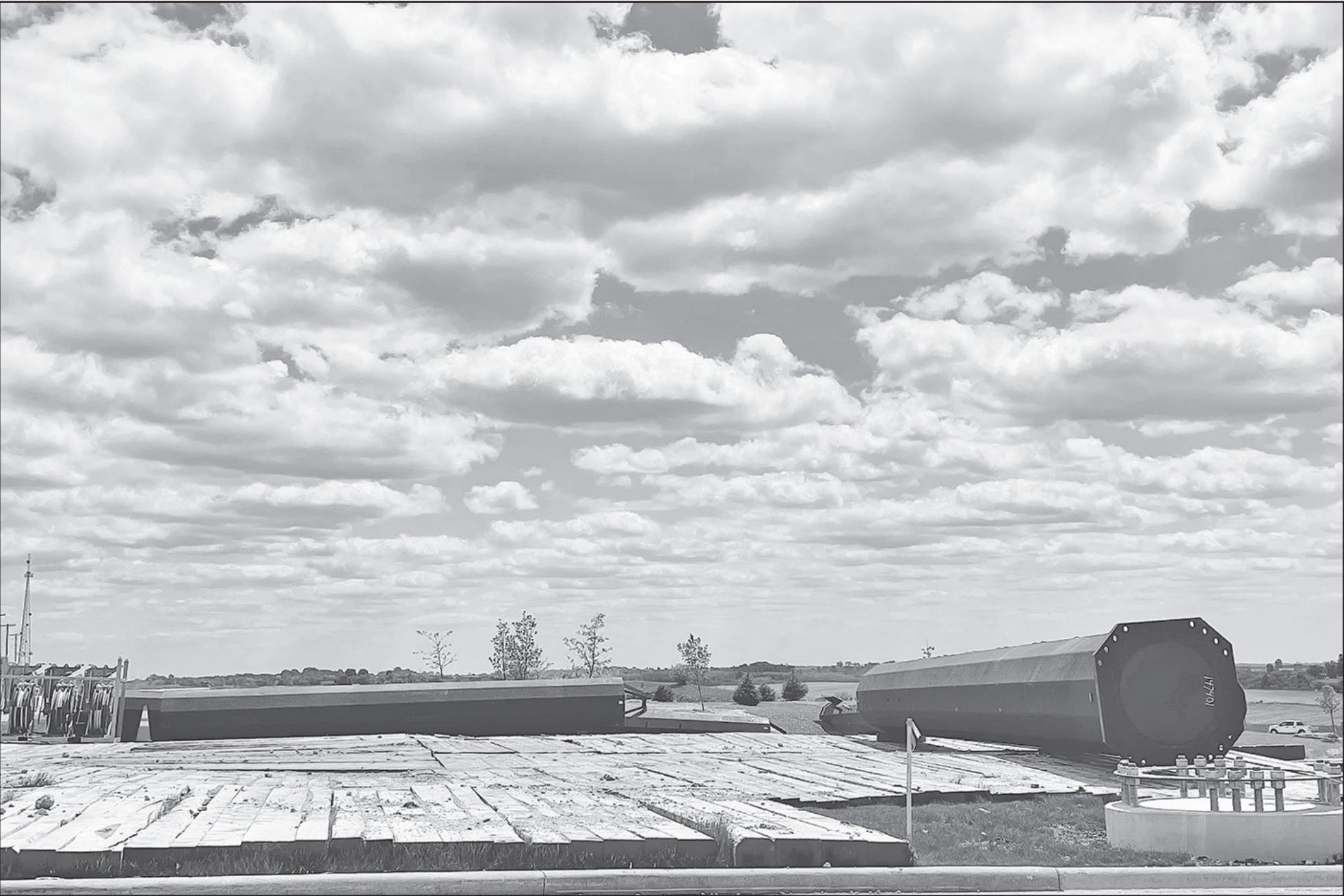
Work continues on the 102-mile, 345-kV transmission line, which is expected to be completed by September 27, 2024.
